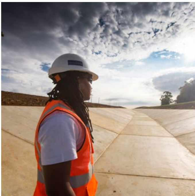
River diversion at Isibonelo Colliery, South Africa
