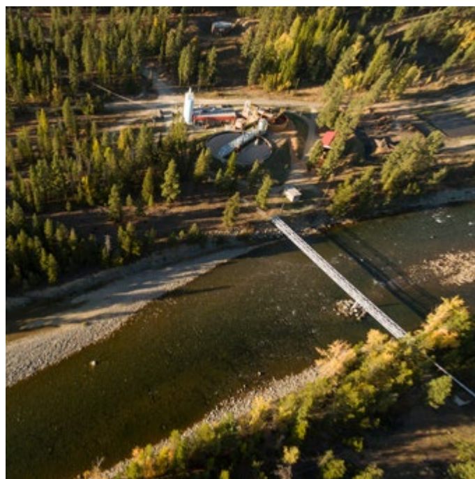
Water treatment plant at closed Sullivan mine, Canada
