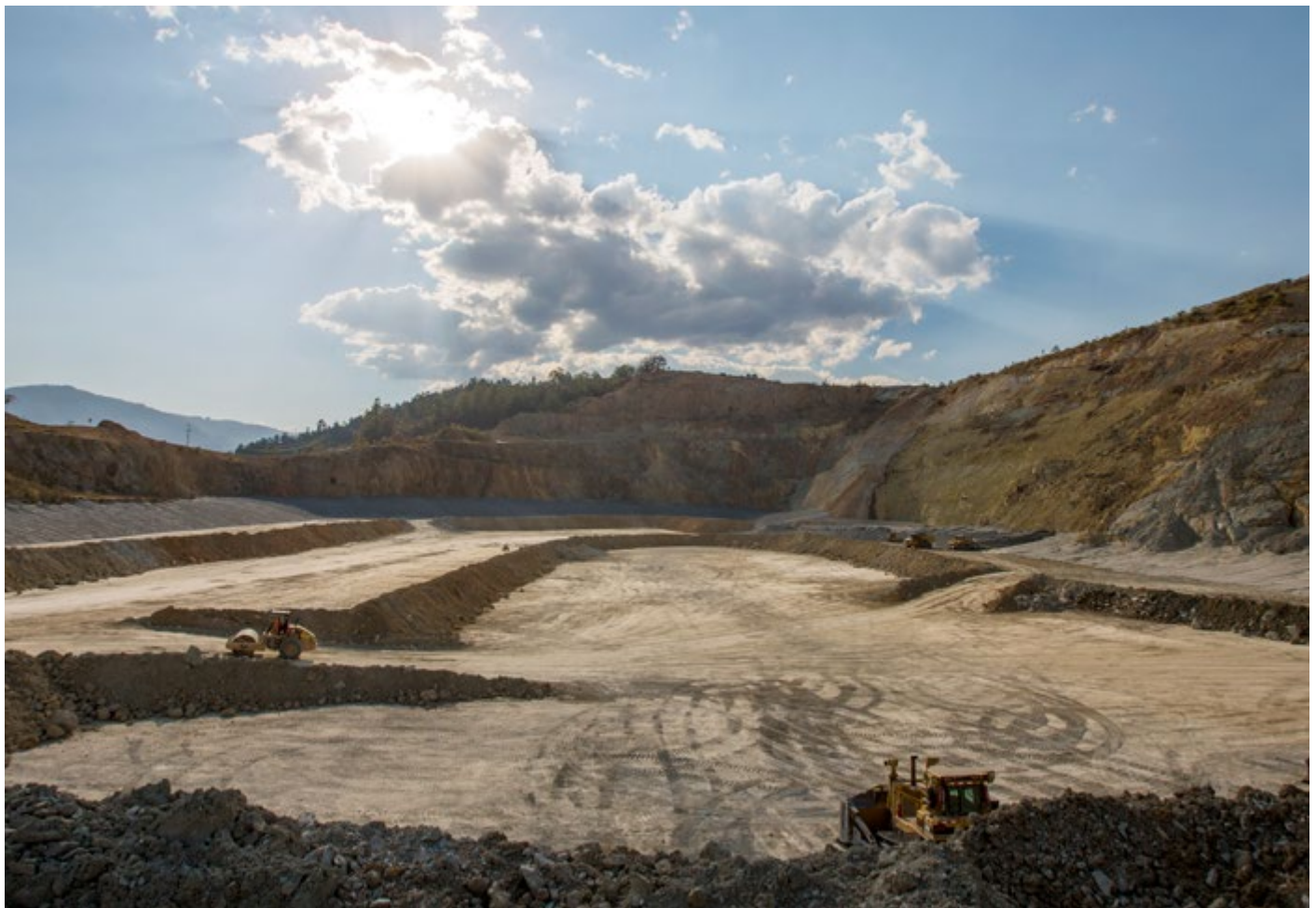
Open pit backfilling at Marlin Mine, Guatemala
