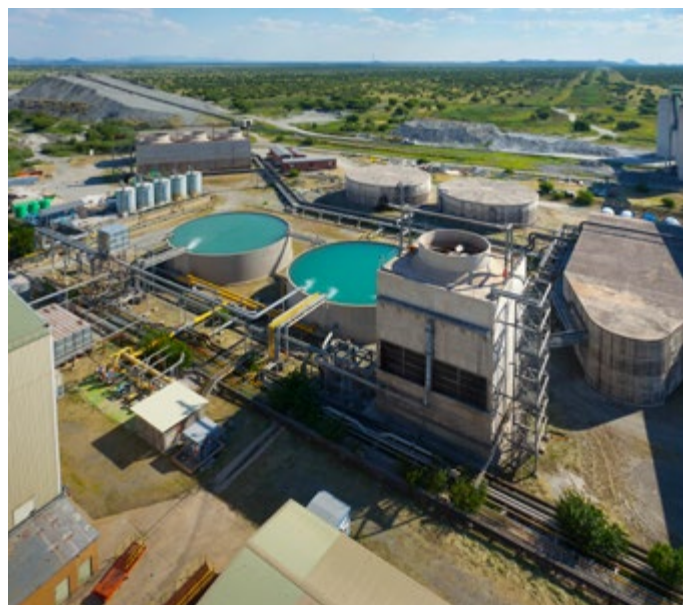
Dishaba mine infrastructure, South Africa
